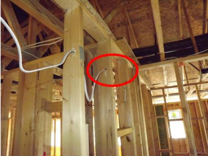
Missing stud guards at master bath.
