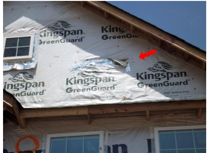
Loose tape / house wrap at front.
