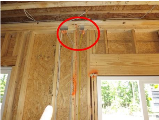
Missing stud strap near rear sliding glass.
