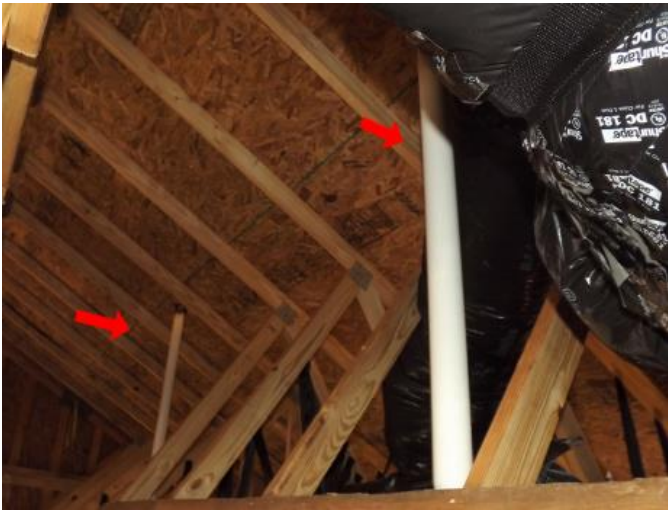
Plumbing vent pipes.
