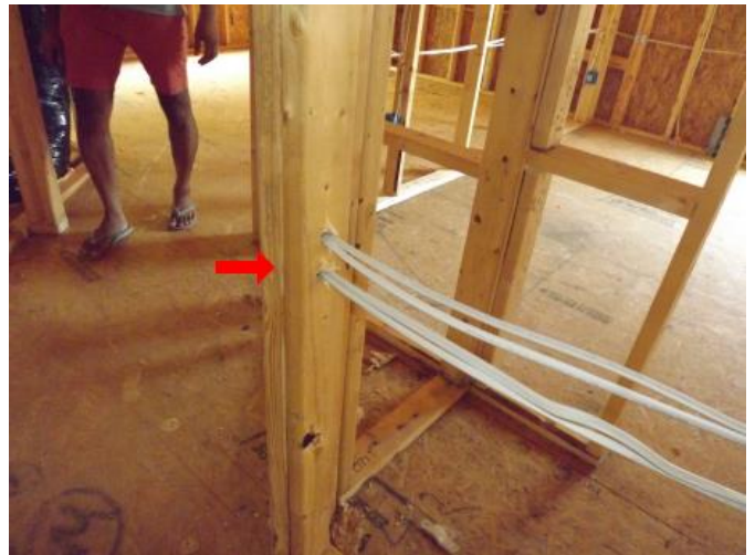
Missing stud guards at second floor hallway.
