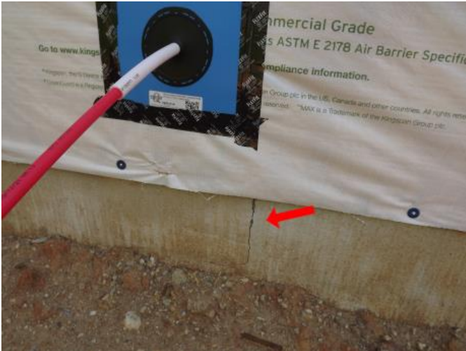
Crack in foundation wall at Left side.
