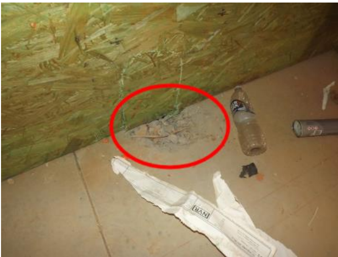
Damaged concrete at kitchen.
