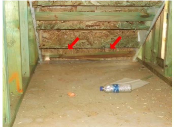
Cracked / damaged support at underside of stairs.
