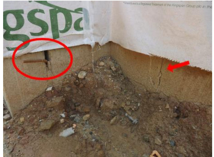
Cracks in foundation wall at rear. Exposed sill anchor bolt.
