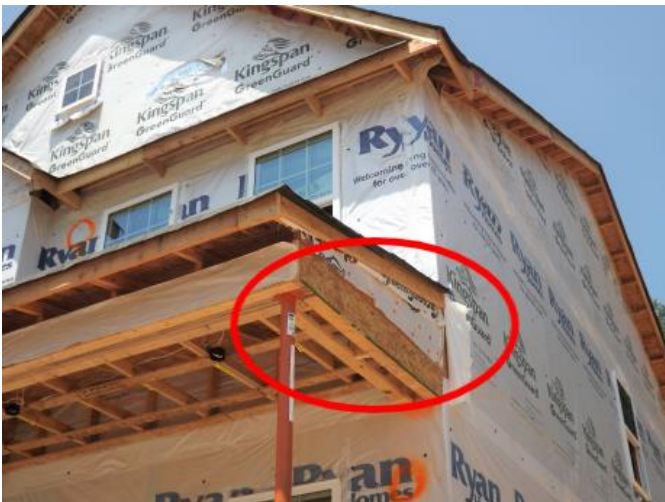
Missing / loose house wrap at Right side.
