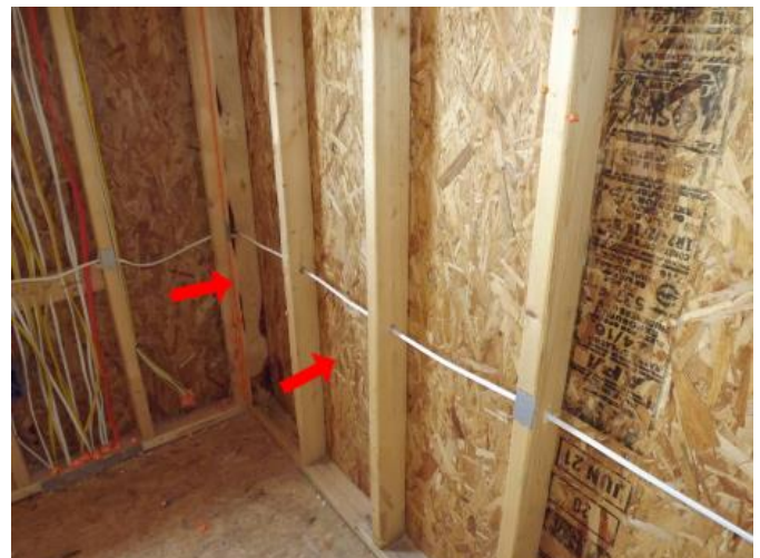
Missing stud guards at second floor loft.
