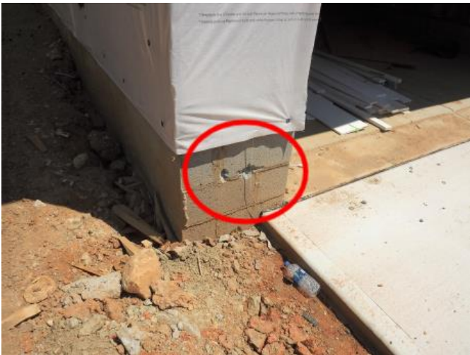
Damage at CMU block to Left of garage.
