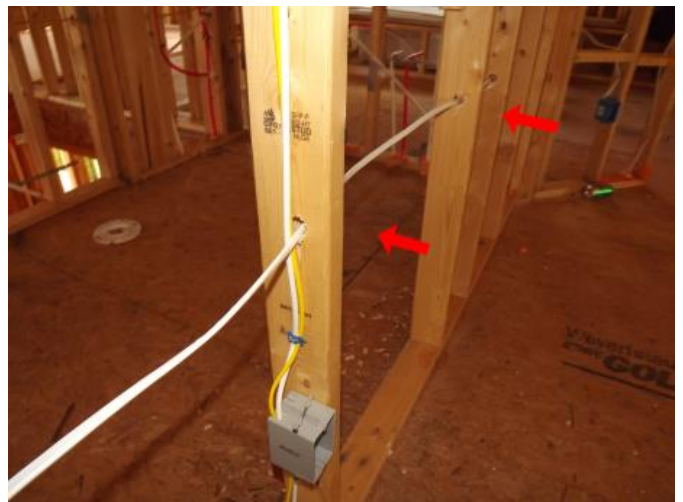
Missing stud guards at master bedroom.
