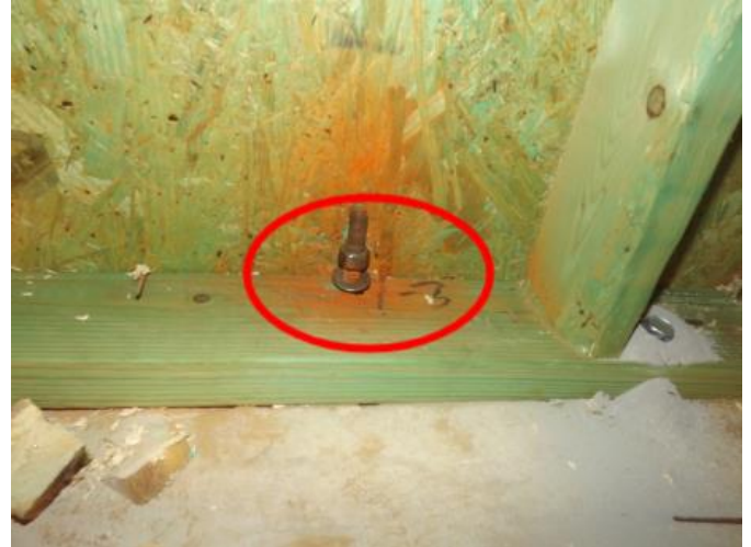
Loose sill plate fastener at kitchen.
