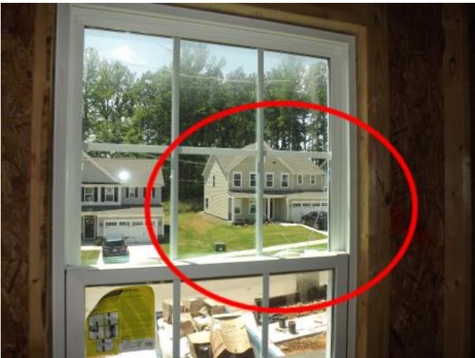
Cracked window at second floor.
