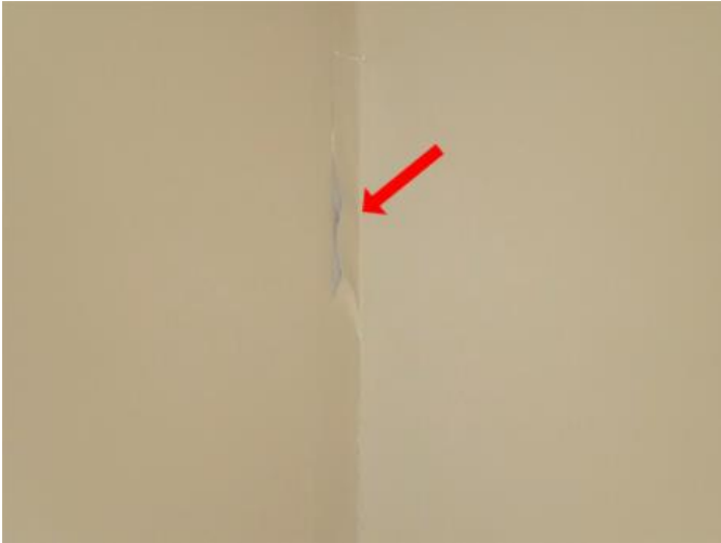
Cracked/loose drywall tape.
