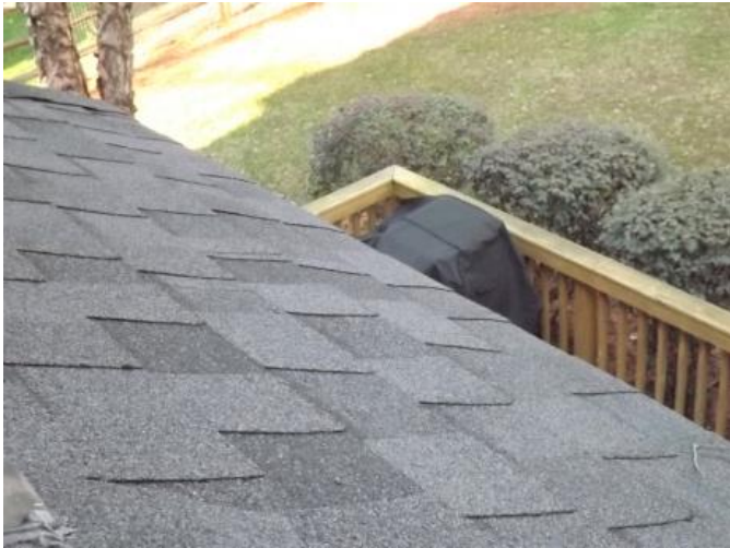
Damaged shingle(s)
