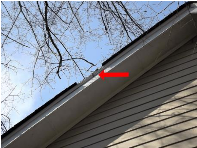
Damaged shingle(s)
