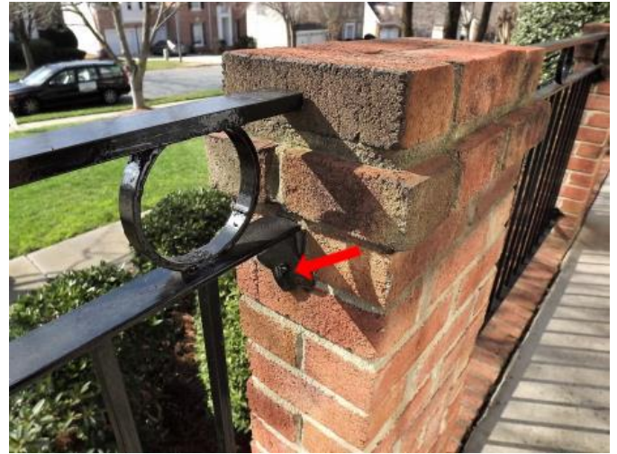
Loose railing bolt
